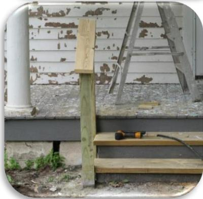
❖ **Paint** used in homes or apartment buildings before 1978 may contain lead. **Chipping paint** inside or outside of the home is harmful. **Dust** can result from paint peeling and crumbling - also if a home is being renovated or if walls are resurfaced.
